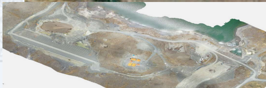
Presa de Taypichaca Avance: 28,91%
